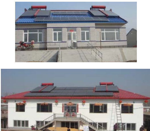
Figure 4. Household type micro-grid heat-electricity combined system
